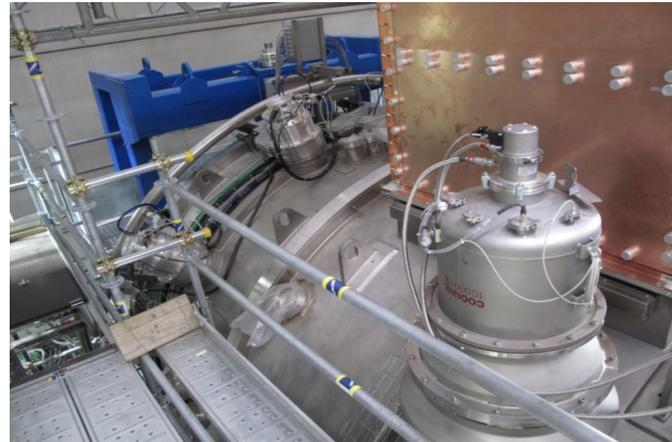
Turbo pumps and cryo pumps installed just outside of the SPIDER Vacuum Vessel
