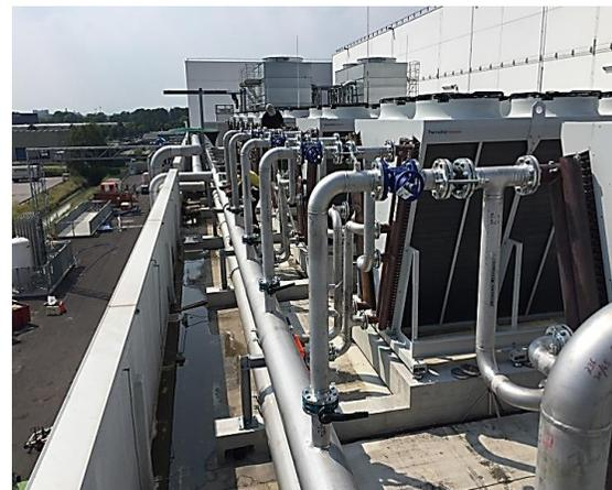
Air coolers and cooling towers installed on the roof. Total power dissipated: 17MW
