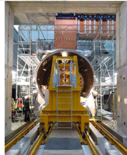
Installation of SPIDER BS inside vacuum vessel
