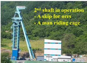
Handeok has two shafts for mining  $1^{st}$  shaft  $\sim 300$  m deep  $2^{nd}$  shaft 600 m deep (NEW)
