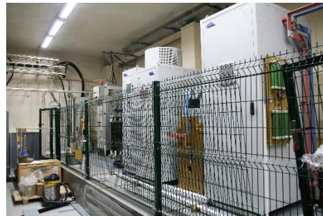
Primary line rectifier 3kV, 3 MW
