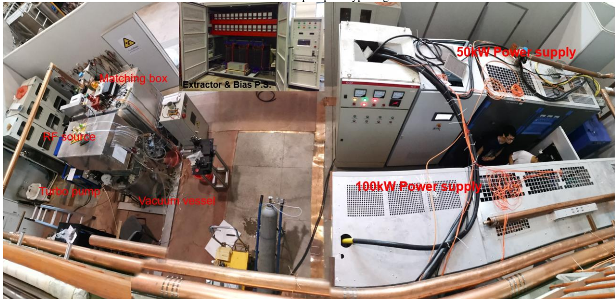
FIGURE 2. The picture of RF beam source test facility
