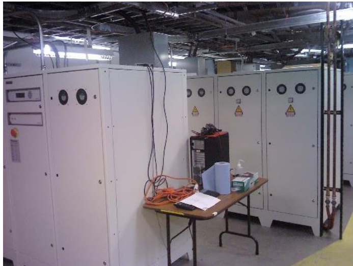
Power supplies for dipole magnets from our subcontractor Danfysik
