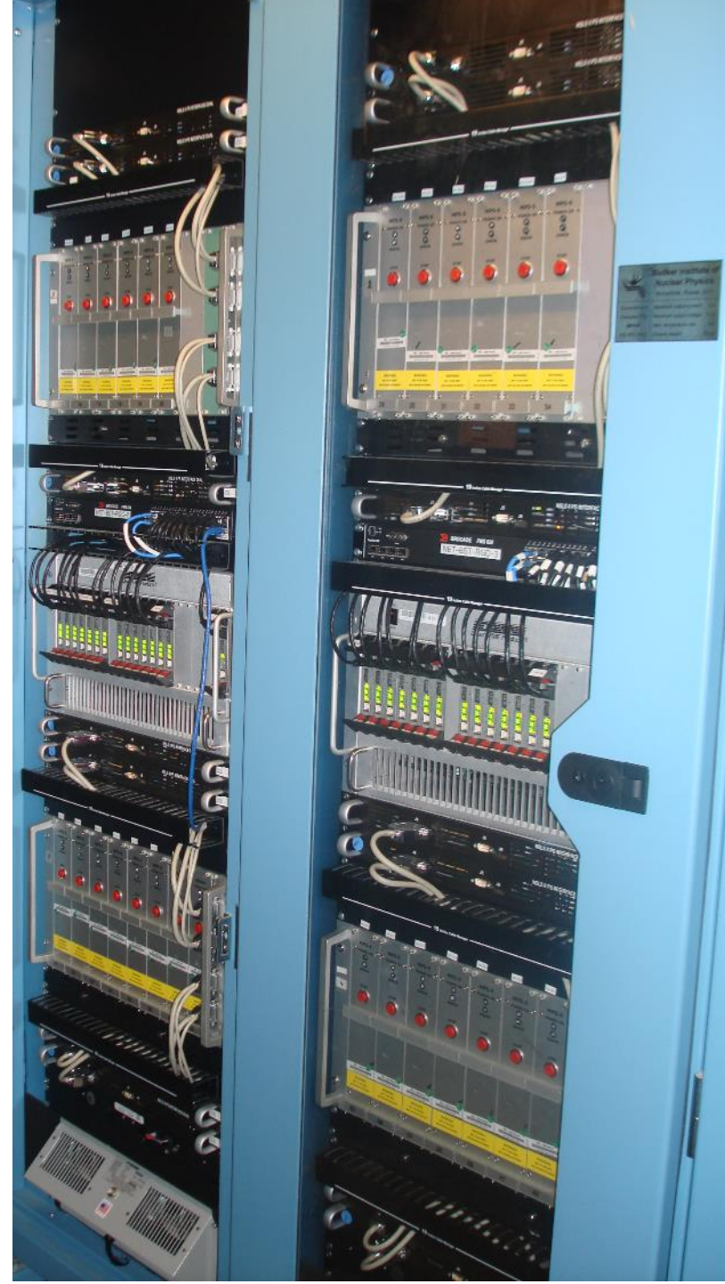
MPS6 – 8 channel crate for corrector and sextupole magnets
