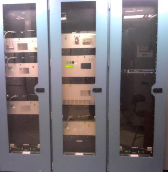
Power supplies for DC septum and quadrupole magnets
