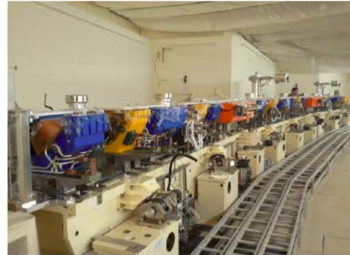
Anchor the 14 m vacuum cell on the girders.
